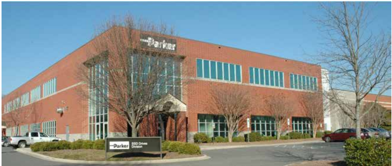
Parker Electromechanical and Drives Division Headquarters - Charlotte, NC
